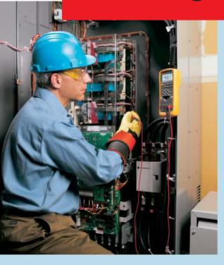
The Fluke 87V DMM overcomes measurement problems caused by the adjustable speed motor drives. These drives adjust the speed of alternating current motors using pulse width modulation that generates a very 'noisy' or 'chopped' signal.
